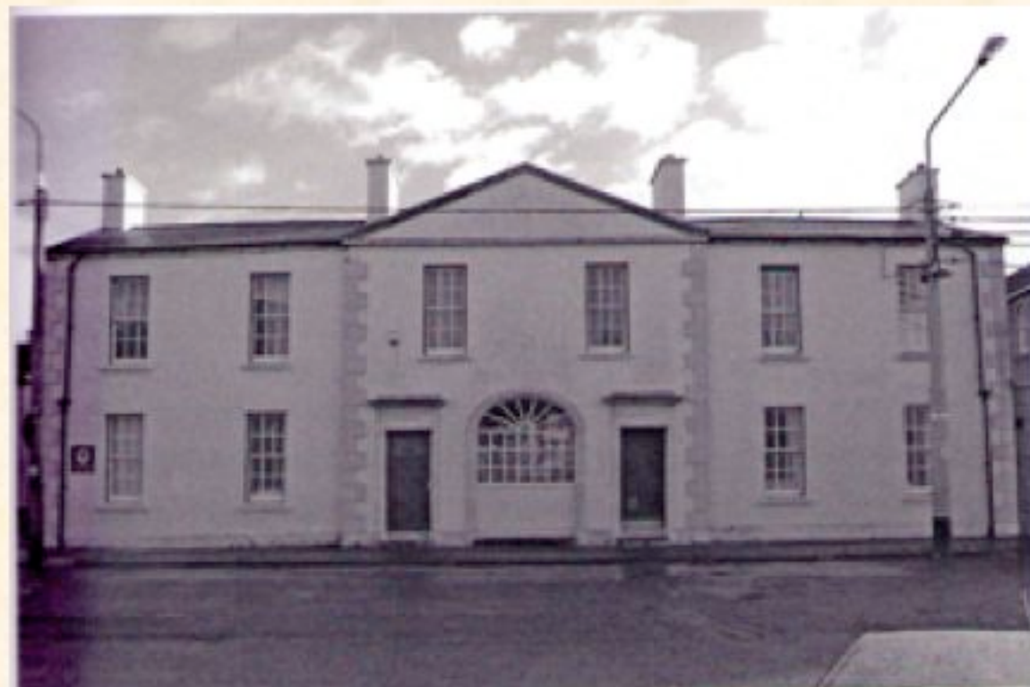
Original Quaker Meeting House on Gratton Street, designed by George T. Beale
